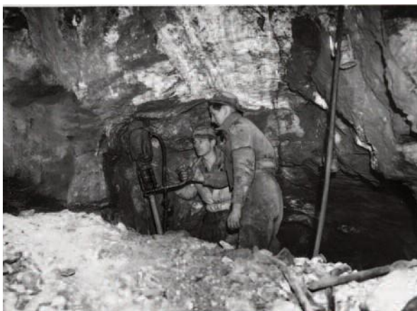
Cowgreen Mine. Miners working underground in a stope in 1949. The baryte vein is clearly seen in the roof: © Friends of Killhope Archive
