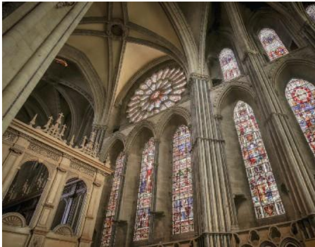
Dark grey cylindrical shafts of Frosterley Marble in the thirteenth-century Early English Gothic pillars of the Chapel of the Nine Altars, Durham Cathedral: Reproduced by kind permission of the Chapter of Durham Cathedral
